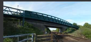
View of Existing Bridges Crossing the York – Scarborough Railway
