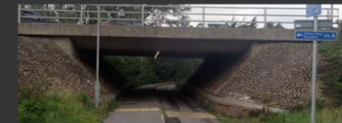
View Through Existing (Western) Haxby Roundabout Underpass
