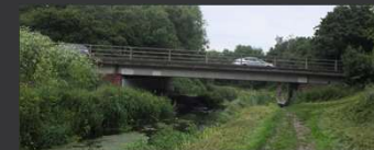
View of the Existing Road Bridge Crossing the River Foss
